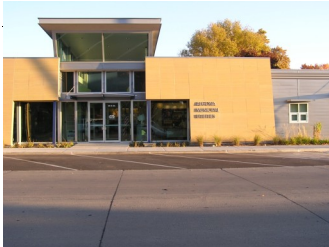
Algonia Municipal Utilities
